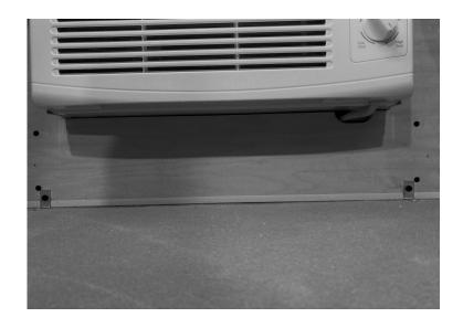
Fasten the angles into the aluminum frame using #10 x 1" flathead sheet metal screws. Reinstall the AC coverboard with the four (4) 1" mounting screws
