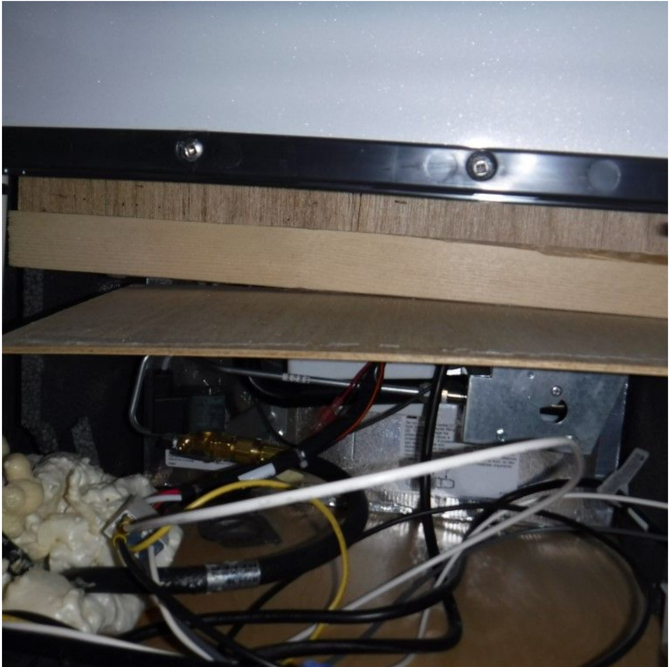
Baffle has broken and fallen down to the bottom of the fridge cabinet
