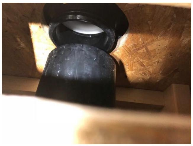
A view from under the trailer right below the shower platform, this is the black tank drain and these are the two pieces that need glued together.
